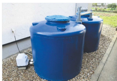
Fig.2 Automatic control rainwater utilization system for detached house
