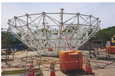
Fig.2 Aperture 13.5m parabolic antenna system (under construction)
