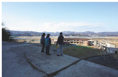
Fig.1 Disaster damage investigation
