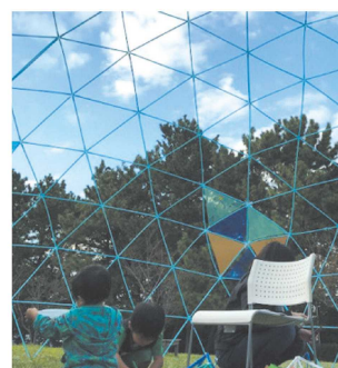
photo.3 Strodome with a diameter of 5 m
