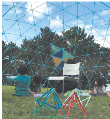
photo.2 Strodome with a diameter of 5 m
